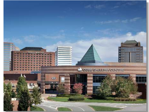
Cobb Galleria Centre Atlanta, Georgia
